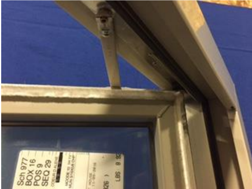
3411 Casement – Open, Hinge Track, Weatherstripping
