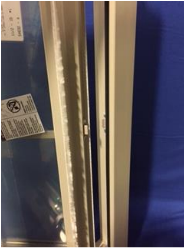
3411 Casement – Open, Weatherstripping, Snubber
