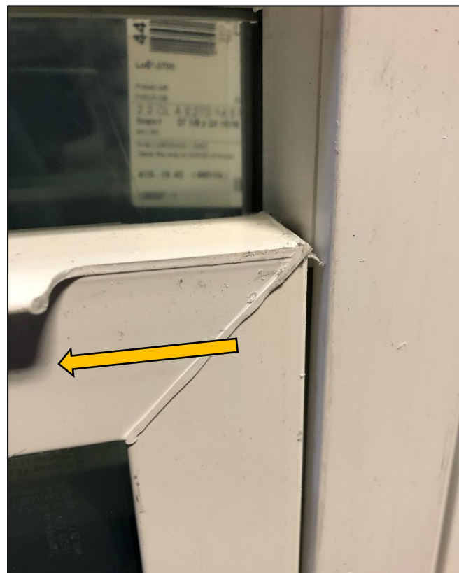
Sash slid to the left, then removed
