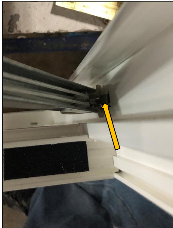
Balancer end with hook (#1)
