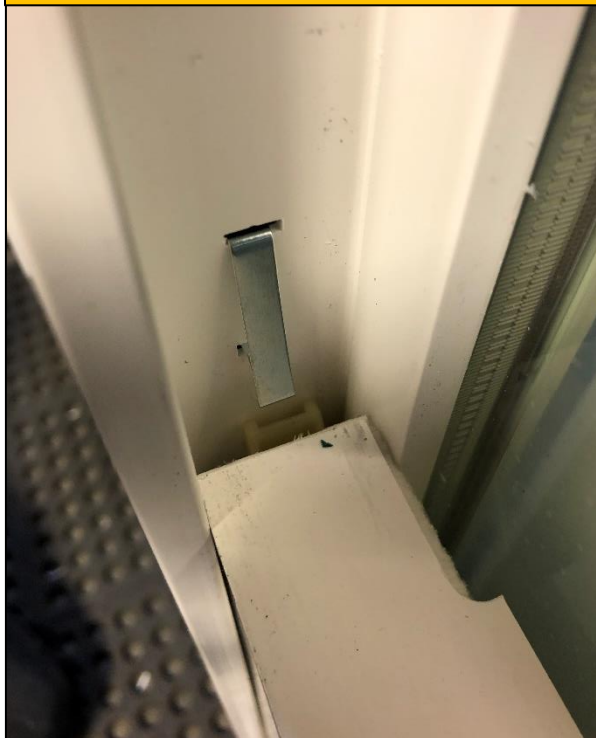
Metal clip engaging the balancer (#1)
