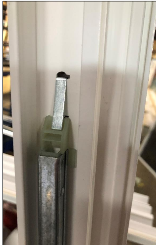
Balancer hooked on clip (#1)
