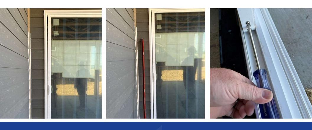
When adjusting the wheels, you want to bring the sash over next to the frame and check the gap or reveal between the sash and frame.
