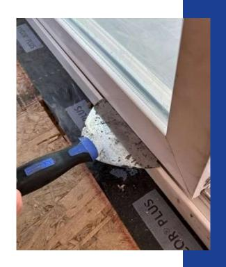
**Left:** When taking the patio door sash out or putting it in, a putty knife can help get the wheels over the mainframe.
