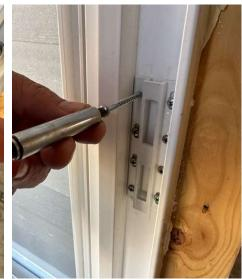
If the patio door sash is not going into the mainframe easily, you will need to check that the frame and sash are straight. There is metal reinforcement inside both sides of the sash and the center fixed interlock. Sometimes, during shipping, the internal metal can get slightly bent from strapping the door into the truck. It is normal to pull or pry on either side of the sash or fixed interlock to bend those back straight.
