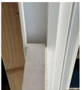
Bottom: You want to raise the wheel/sash, so it is not dragging on the slider track. Check the top and bottom of the sash and confirm the weather strip is still making good contact with the frame.
